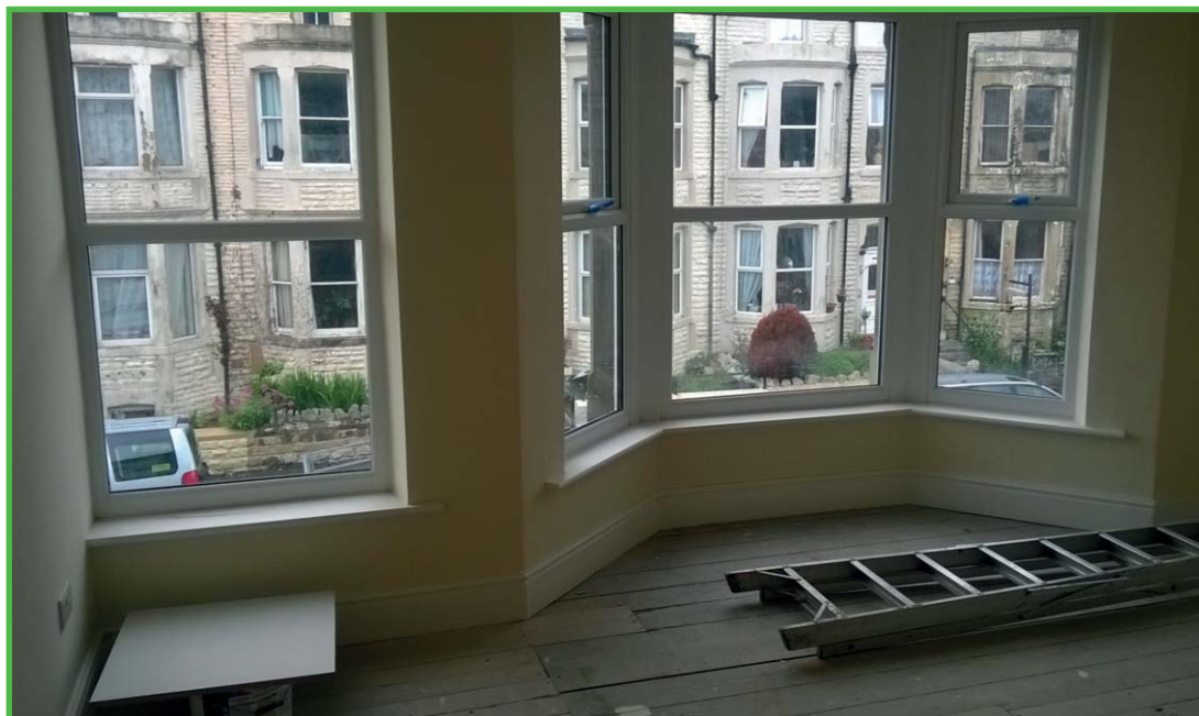
Left: House refurbishment in progress by Methodist Action North West
