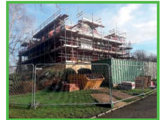
Above: Denehurst House during refurbishment by Groundwork (GM)
