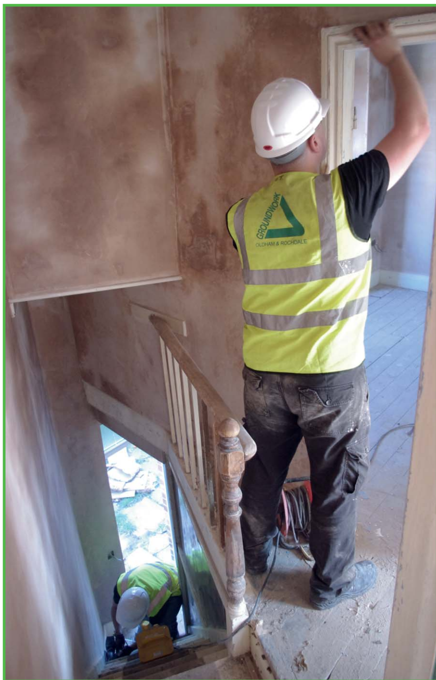
Above: Refurbishment work by Groundwork (GM)
