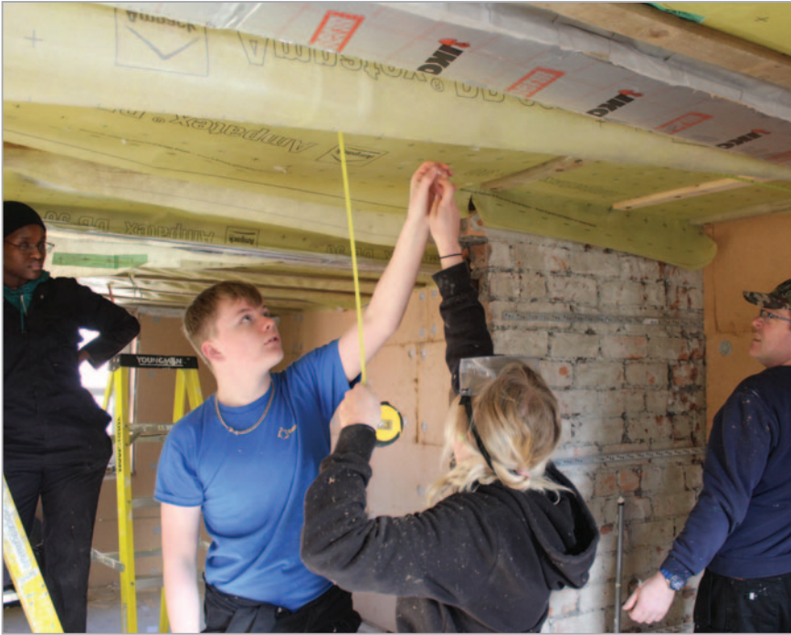
Canopy Housing trainees installing vapour barrier
