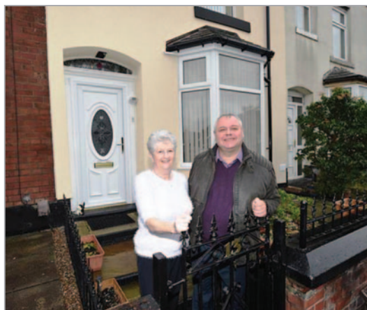
External wall insulation in Rochdale
