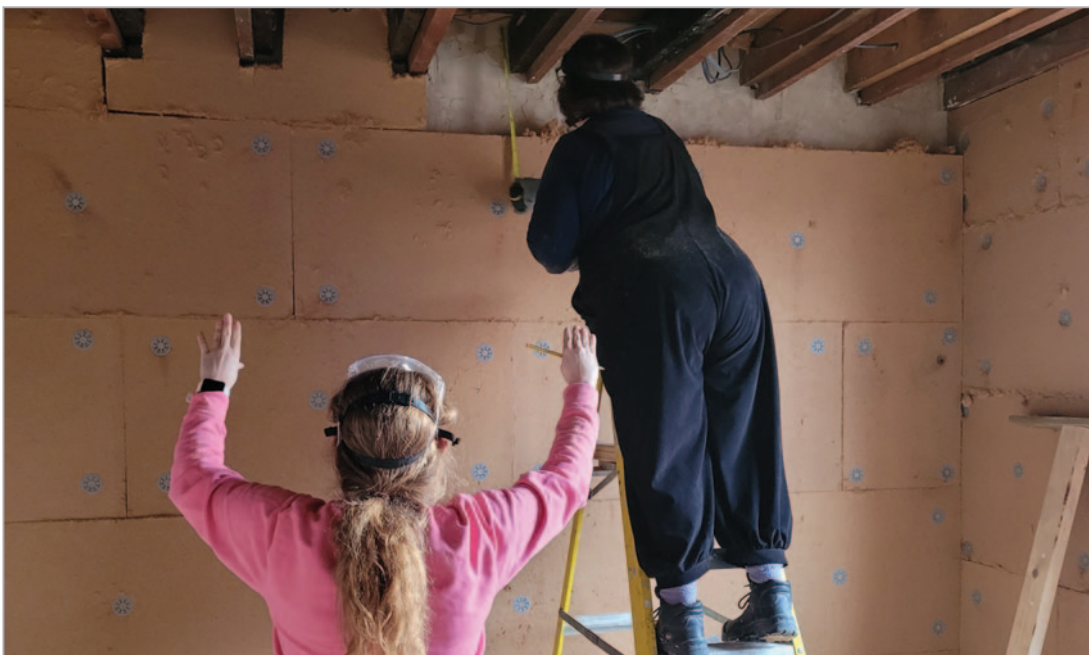
Canopy trainees install wood fibre insulation
